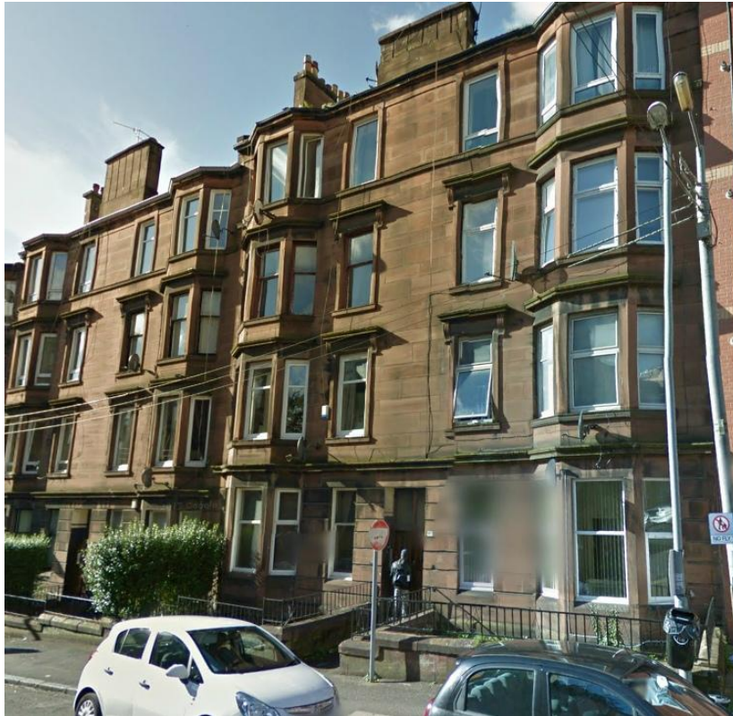
Figure 4-4: Home 2 as viewed from the street at the front of the building.
